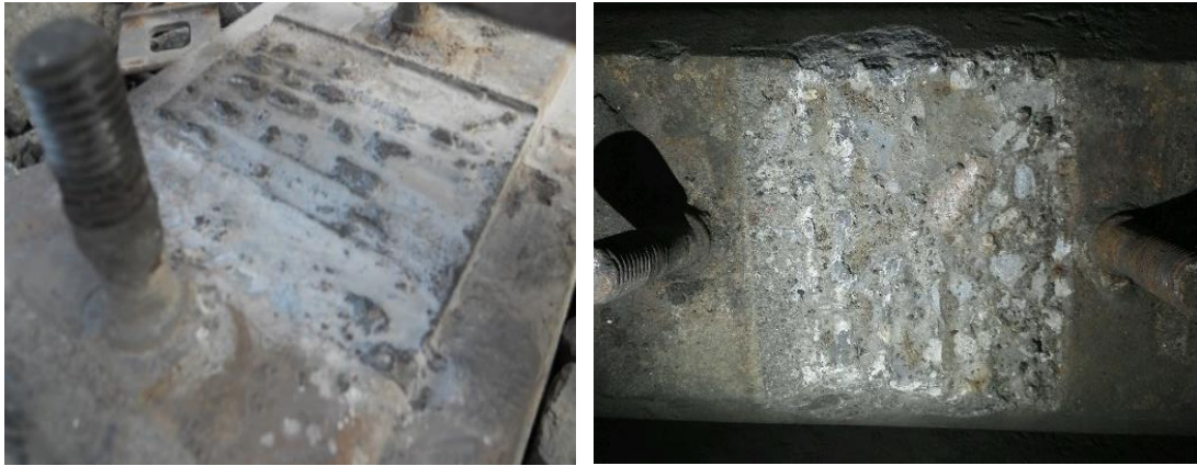
Fig. 2. Typical RSA of prestressed concrete sleeper
