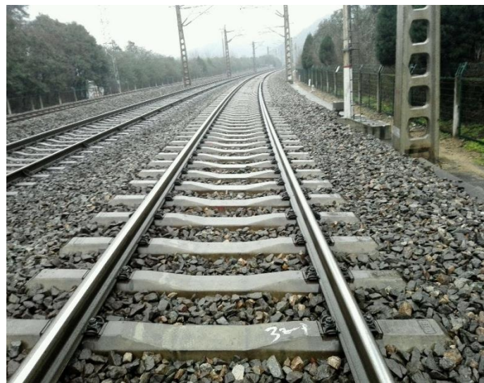
Fig. 1. Prestressed concrete sleepers in ballasted railway track
