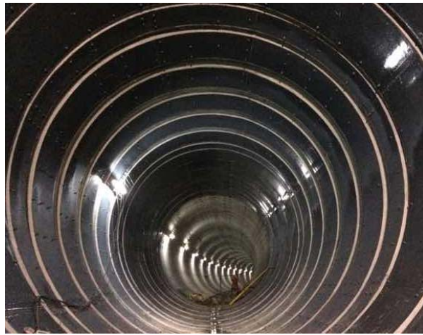
Figure 1 Photograph of a steel plate reinforced segmental tunnel lining
