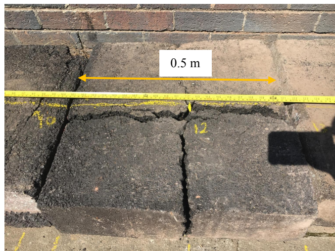
Figure 2: One of the tested asphalt slabs
