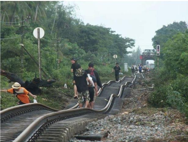
**Fig. 4.** Track condition after a flash flood in 2016 (Courtesy: State Railway of Thailand). Concrete sleepers have ability to retain to certain extent the original alignment and geometry. However, it is important to note that replacing timber with concrete sleepers without improving ground condition can pose a significant georisk of formation failure and differential track settlements under various climate uncertainties such as high intensity rain, flooding and sea level rise.
